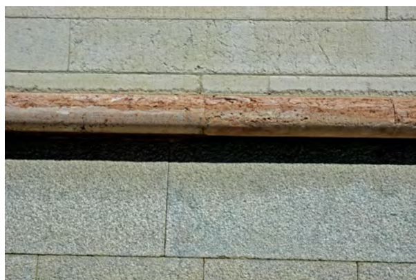
Tandhuggen kalkstenslist, kryssharnad granitsockel, Strandvägen, Stockholm
