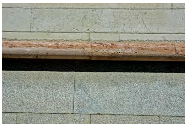
Tandhuggen kalkstenslist, krysshamrad granitsockel, Strandvägen, Stockholm
