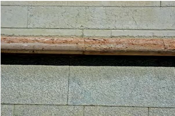
Tandhuggen kalkstenslist, krysshämrad granitsockel, Strandv 33
